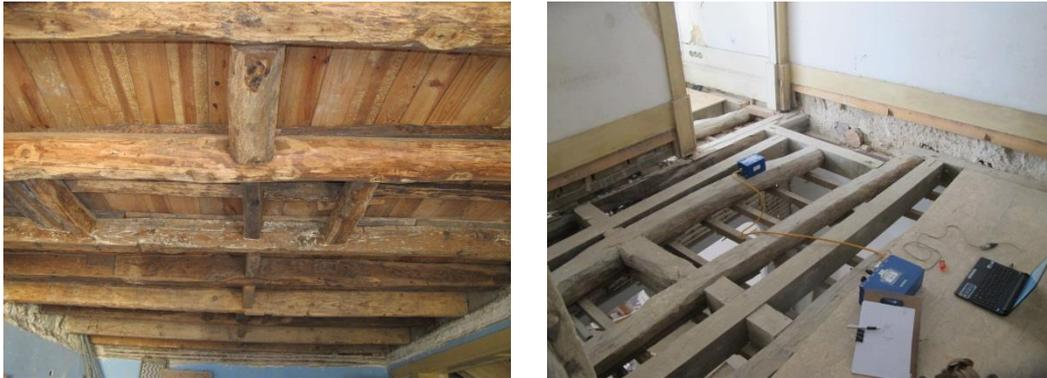
Figure 1 – Timber floors: a) timber beams and wooden floorboards; b) performed tests.
