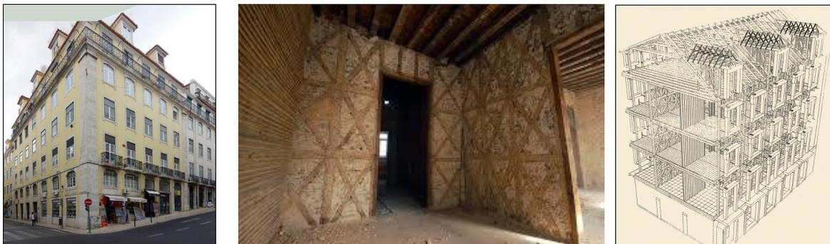
Figure 1 – A combined masonry and timber structural traditional system used Lisbon, Portugal
