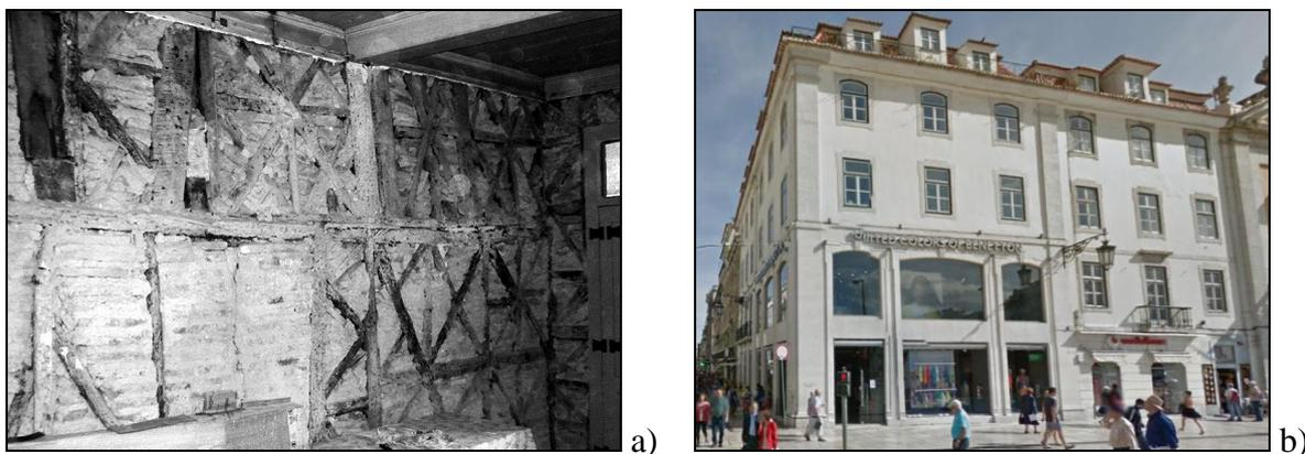
Figure 2 – Traditional “Pombalino” buildings in Lisbon: a) removal of a masonry wall, replaced by a steel H shape steel beam; b) total rebuilding of the first floors to create a commercial open space producing the masonry wall-piers discontinuity on both façades of a “Pombalino” corner building.
