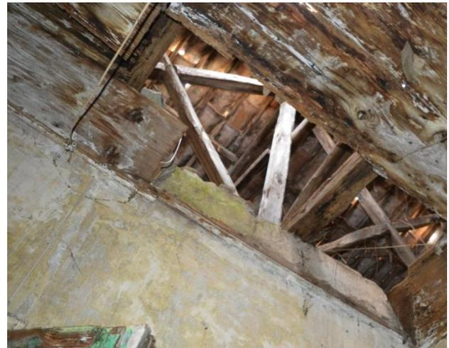
Fig. Timber frame emphasizing alternated notches at the ring level (on the left) roof Saint Andrew crosses (on the right)
