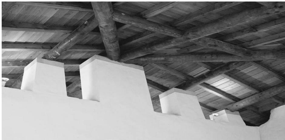
Fig. 3 – The timber roof structure with the short masonry pylons supports.
