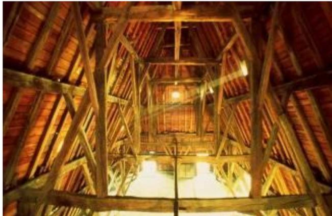
Fig. The timber roof structure of the north-east tower nowadays (photo C.B.)
