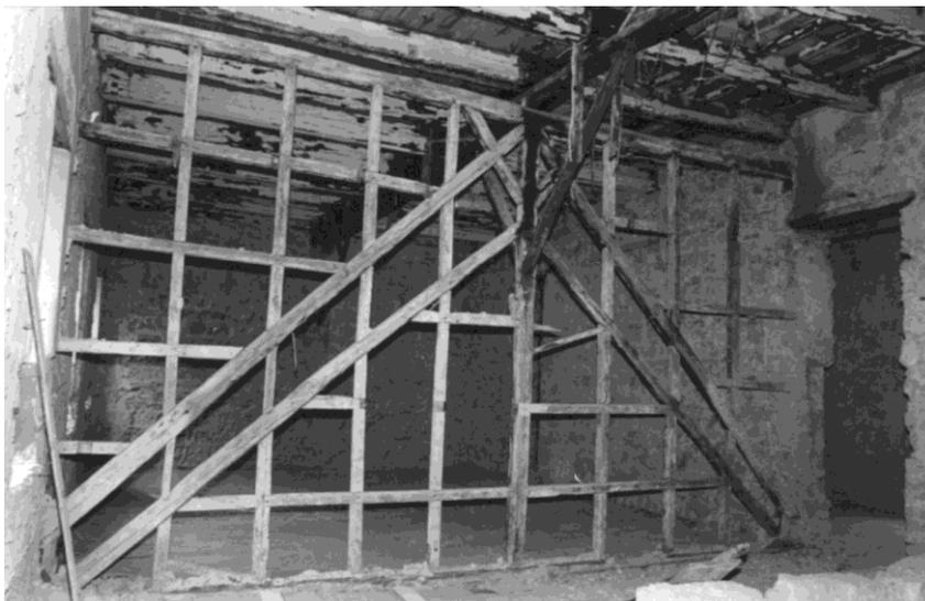
Wooden systems for ceiling support and lintel of openings and lighten partition wall.
